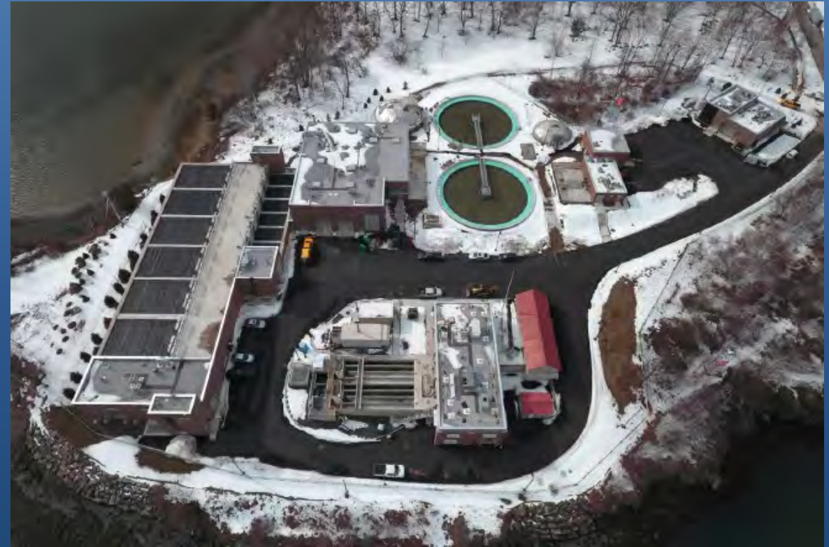
Sewer – Peirce Island Wastewater Treatment
